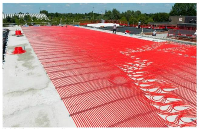
Fig.2 Build-up of the energy roof
