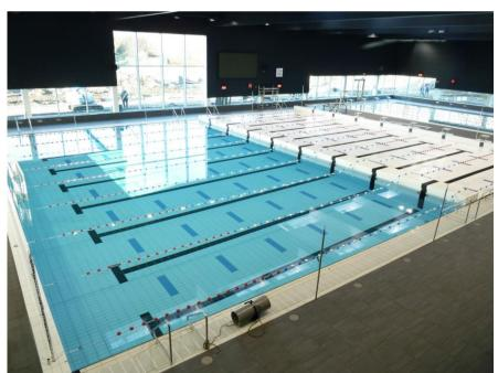
Fig. 1 Nekkerpool inside view, showing the swimming pools with adjustable floors
